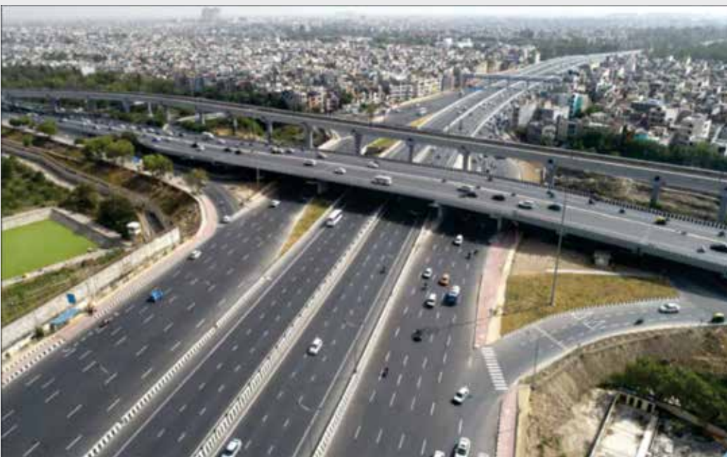
14 Lane Delhi-Meerut Expressway
